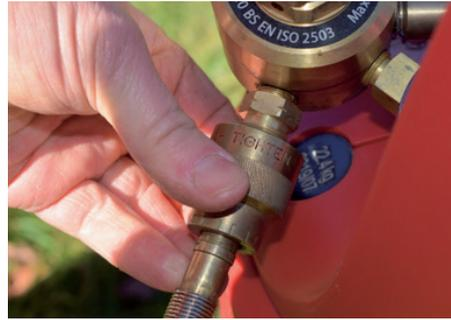
Check that the connection hose to your application has an O-ring and then connect to the outlet of the regulator, again by turning the nut anti-clockwise.
